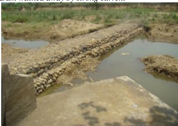
Dam constructed with Sausage wire & boulders
